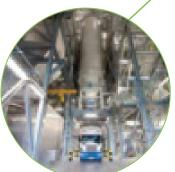
**3.** Compressed air pulses shake off the APCR into silos. The APCR is removed from the site by road tanker.
