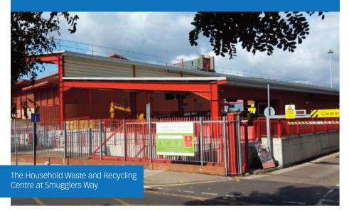
The Smugglers Way HWRC is based on a split-level concept, so that the public is physically separated from the operational activities. This layout provides greater flexibility to users when they deposit material and has reduced waiting times. This, combined with a significant increase in the number of cars able to queue on site at peak times, has helped to reduce local traffic congestion.
