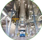
3. Compressed air pulses shake off the APCR into silos. The APCR is removed from the site by road tanker.
