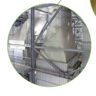
**4.** Clean hot gas is drawn out of the fabric filter bags through a heat exchanger which allows heat to be transferred from the gas into the boiler feed water.
